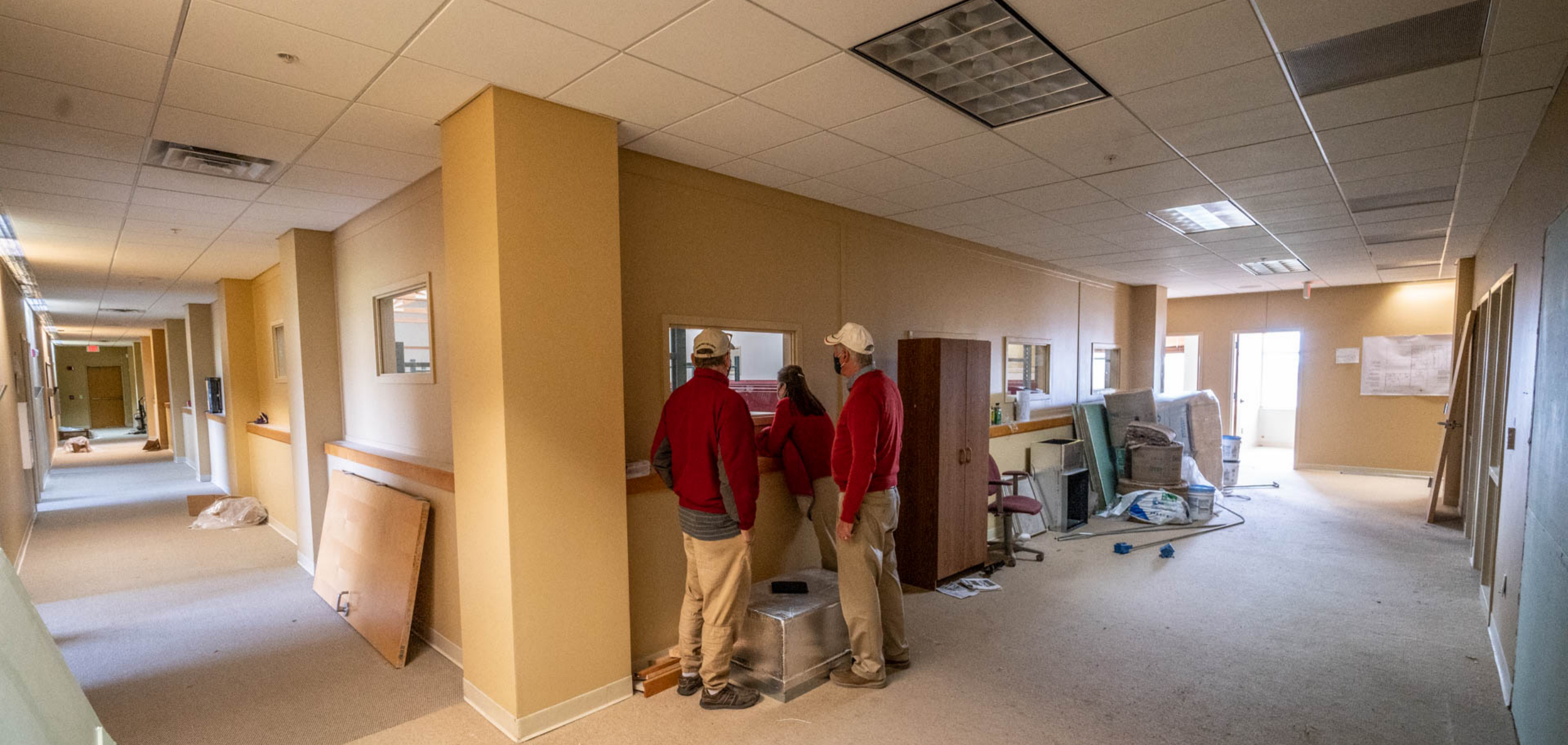
North Wing – new dorm rooms in the making
